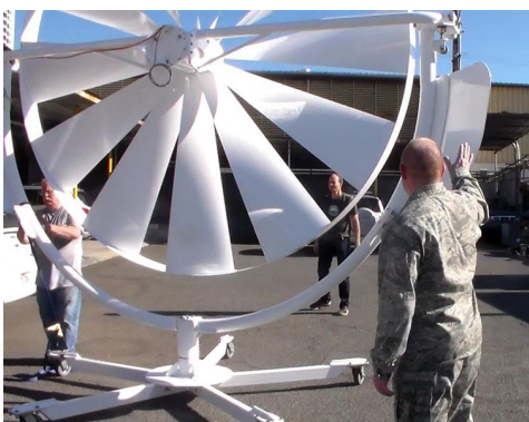
ENERGY HARVESTING TECHNOLOGY Natural Power Concepts personnel and the AFRL Materials and Manufacturing Directorate inspect the spoke wheel medium wind power system, one of a number of energy-harvesting technologies being installed as part of the five-year, $20 million cooperative agreement with AFRL that will establish a microgrid demonstration project at Joint Base Pearl Harbor-Hickam, HI.
