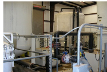
"Pump and treat" system reduced groundwater plume at Reese AFB, TX by 99% since 2004
