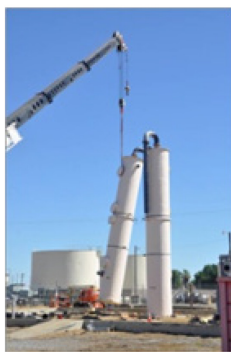
Crane removing first of two air stripper towers, used to treat contaminated groundwater at the former Castle AFB in Atwater, CA
