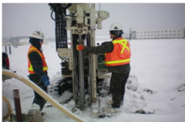
Monitoring Well installation at former Galena FOL in Galena, AK
